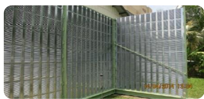
Temporary metal noise barrier
