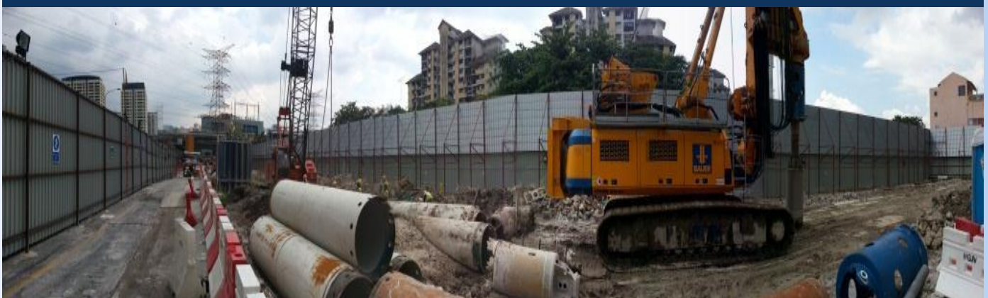
▲ Malaysia KVMRT – Taman Maluri Launch Shaft
