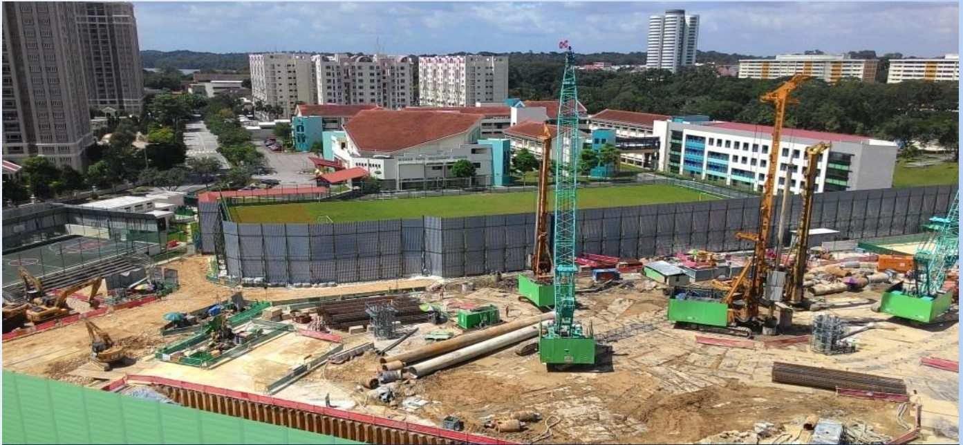
▲ Thomson Line – Bright Hill Station at North Shaft
